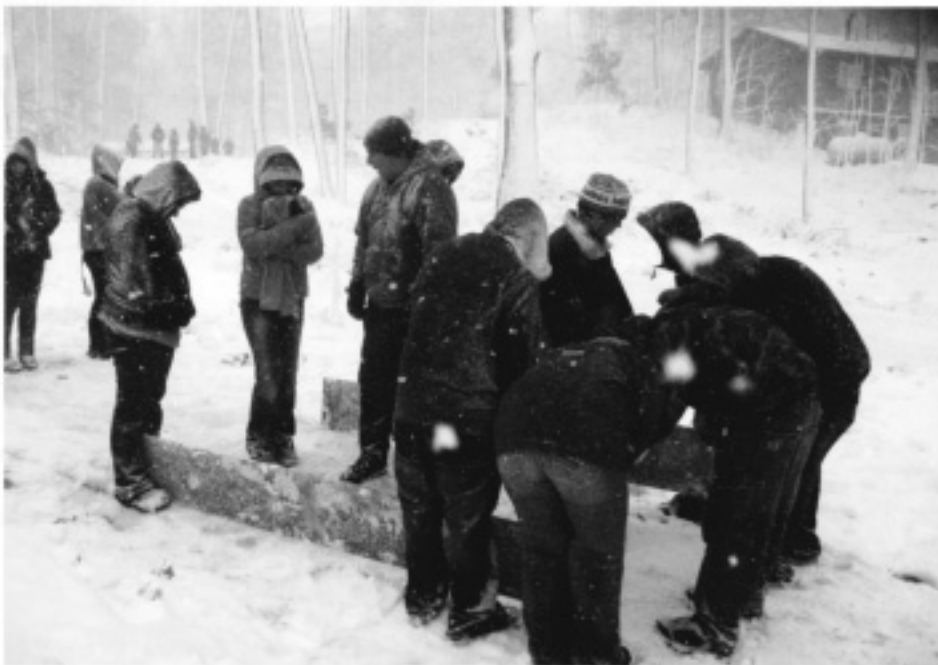
Roger Hatlen (RHS), middle, helps students transfer elevations using 8' lengths of plywood, a plumb bob and wooden folding ruler.
