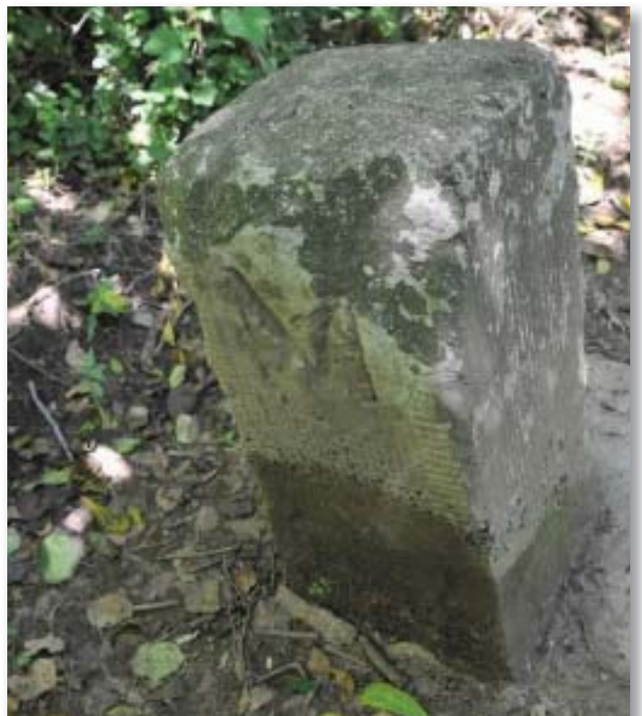
The markers each have an “M” on their southern sides and a “P” on the northern side, to mark the Maryland and Pennsylvania sides of the Mason-Dixon line.
