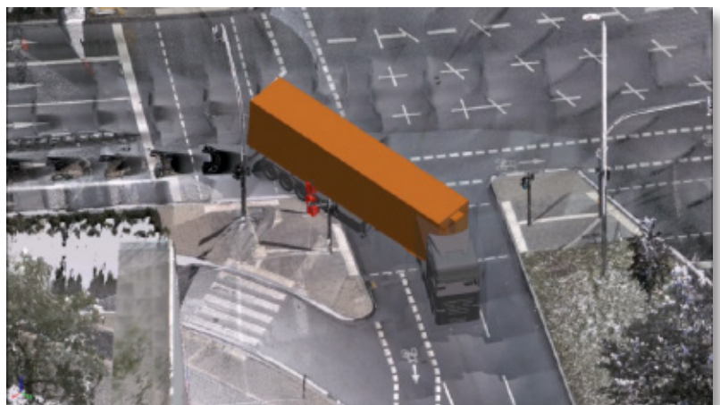
Traffic routes are analysed using digital twins to ensure large vehicles avoid collisions. (Image courtesy: Hexagon)
